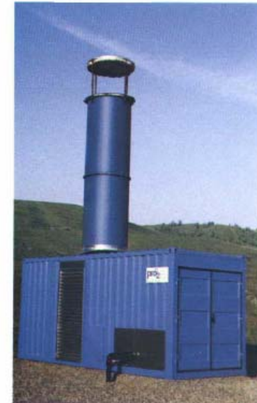
Location: landfill Remo, Belgium Specifications: mobile booster / high-temperature flare unit
