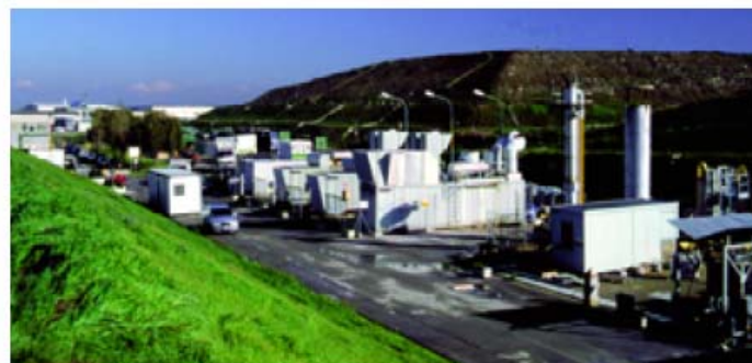
Containerized degassing system with separate rooms for booster, high-temperature flare and monitoring/control facilities.
