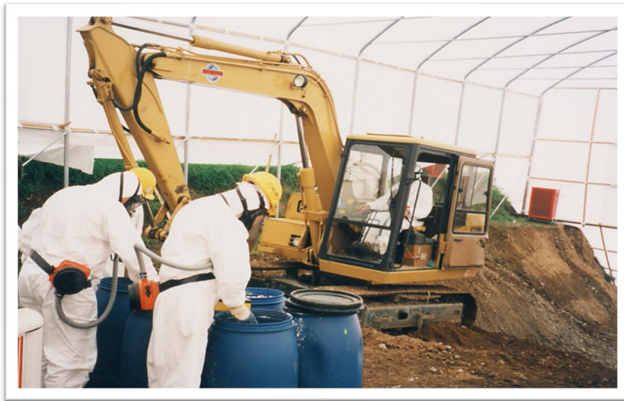
Retrieval of guinea pigs contaminated by ^3\text{H} in the decommissioning of a pharmaceutical factory
